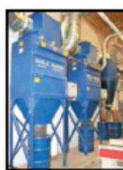
View of Filter 1 "Pulsatron" Dust Collectors
