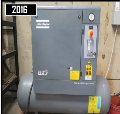
2016 Atlas Copco GX7P EL 10Hp Rotary Air Compressor
