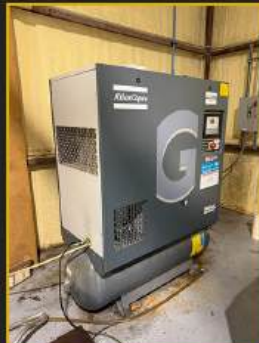
2019 Atlas Copco GA7FF Workplace Air System
