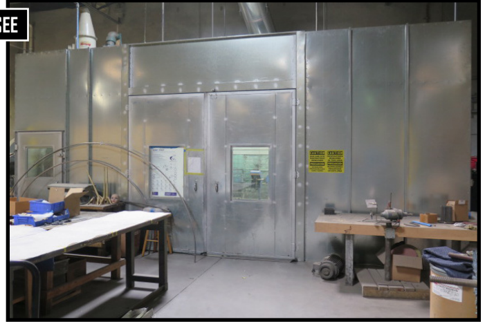
24' x 24' Paint Booth w/ Filtration System and Lighting
