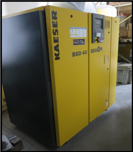
2010 Kaeser BSD40 40Hp Rotary Air Compressor
