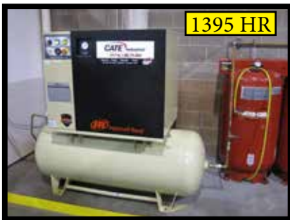
INGERSOL RAND 15 HP ROTARY AIR COMPRESSION
